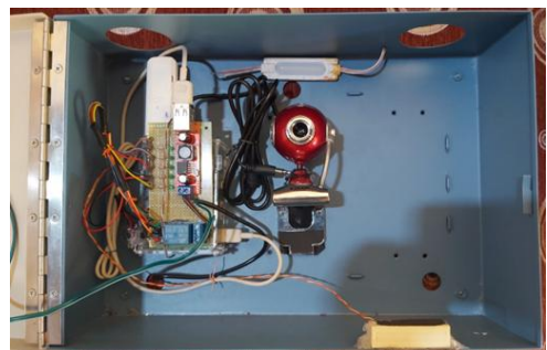
Fig. 4 Installation of the Access control system.
